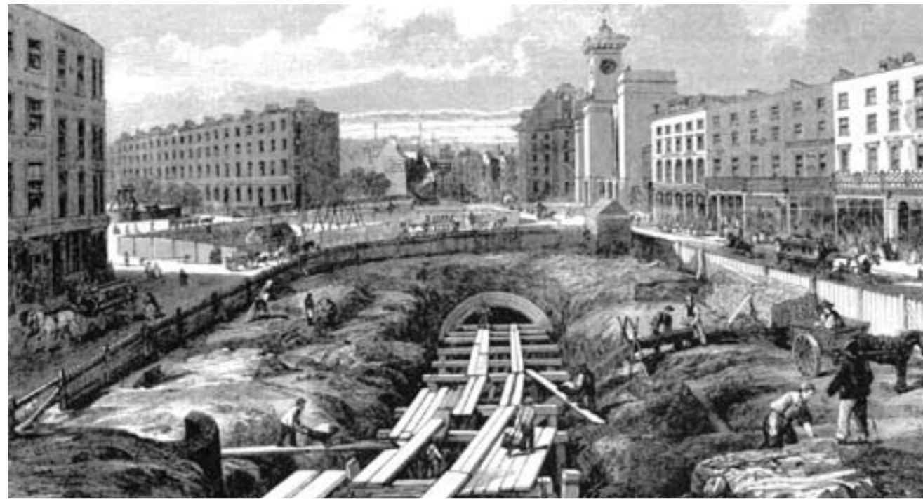
Right: cut-and-cover tunneling for the Metropolitan Railway in 1861; below right: a depiction of King's Cross station on its opening in 1852
